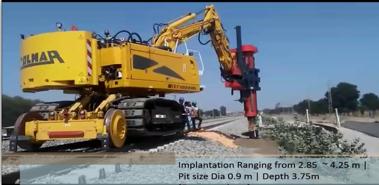
OHE Foundation using Mechanized Auger
