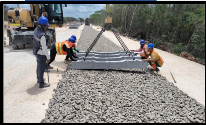
1.- PLACEMENT OF SLEEPERS
