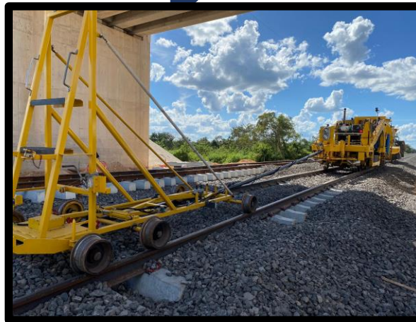
5.- TRACK LIFTING AND LEVELING
