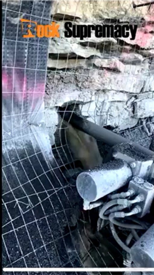
Horizontal Drain Wagoner Slope Stabilization 10/18/2022
