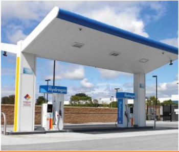
Hydrogen Fueling Stations
