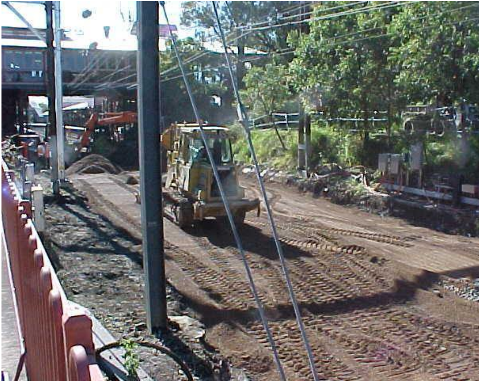
Track Reconditioning Sydney Trains
