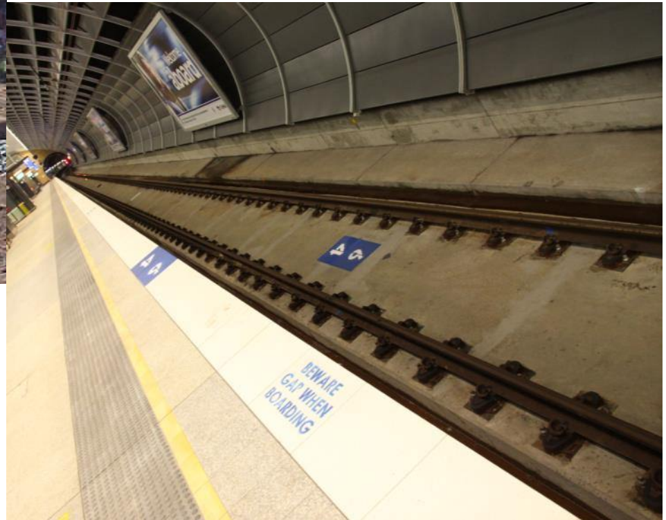
Slab Track Epping-Chatswood Tunnel, Sydney
