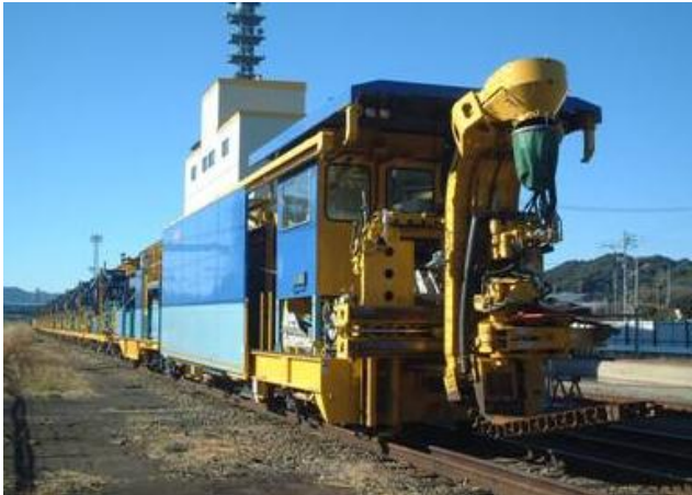
(1) Ballast replacing (Japanese-Made Machinery)
