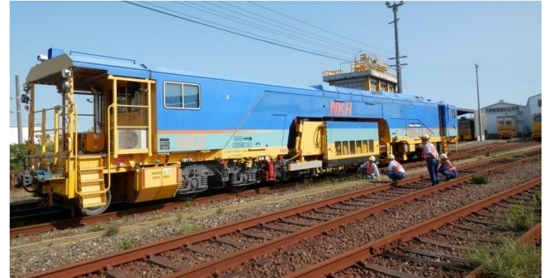
(2) Tamping and correcting track irregularity
