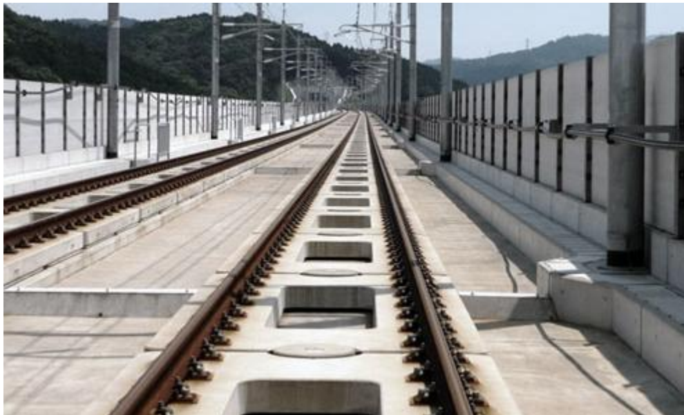
Photo: Japan Railway Construction, Transport and Technology Agency
