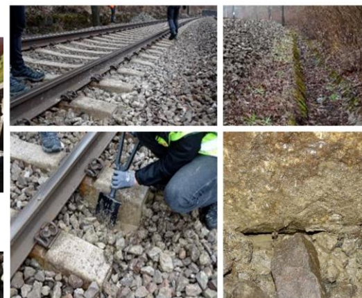
Maintenance: Screw-hole renewal
